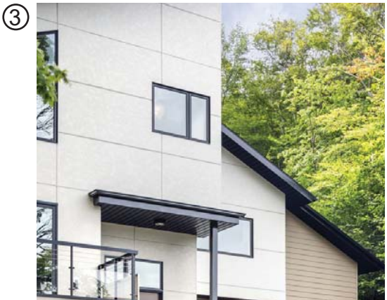
FIBER CEMENT PANELS 2' X 8' AND 4' X 8'
