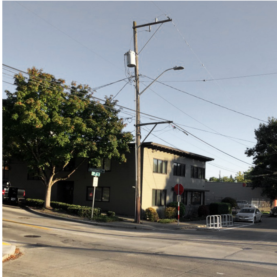
1. Pole and HV Power Line (requires 14' power line setback shown in diagram)
