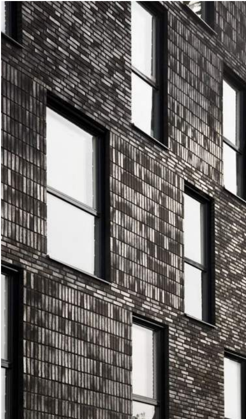
Quality Materials + Detailing - Brick
