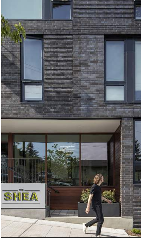
Well Defined Residential Entry
