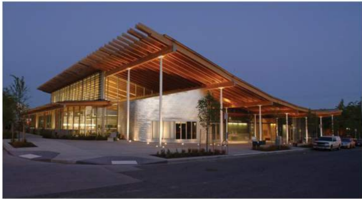
5 BALLARD BRANCH- SEATTLE PUBLIC LIBRARY
