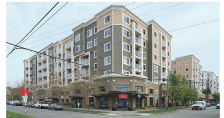
12 BALLARD PLACE CONDOMINIUMS
