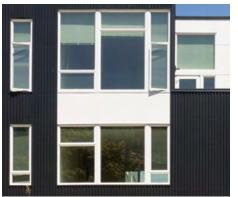
5. WINDOW FRAMES (WHITE) 6. FIBER CEMENT INFILL PANELS (WHITE)
