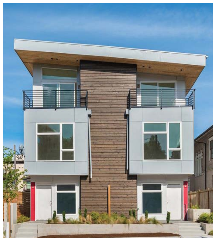
122 17TH AVE EAST
