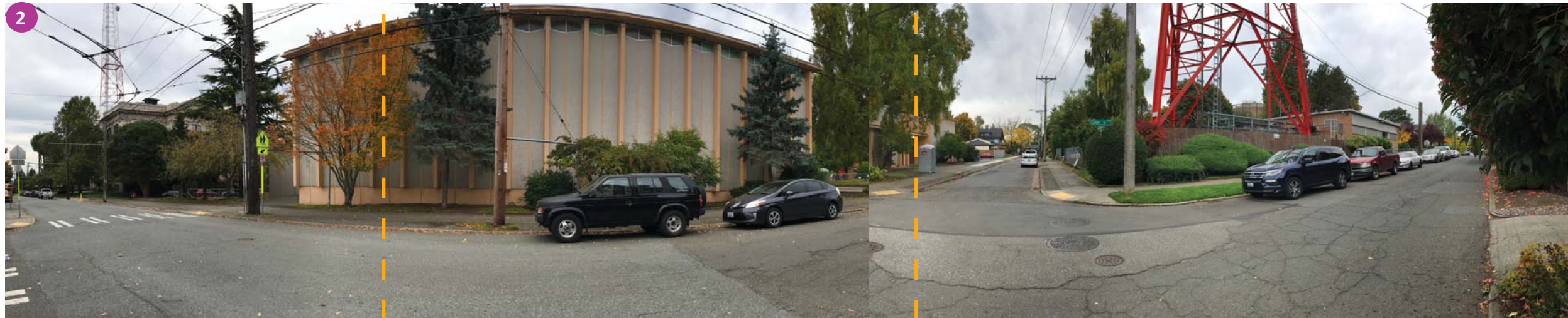
PROJECT SITE OPPOSITE
