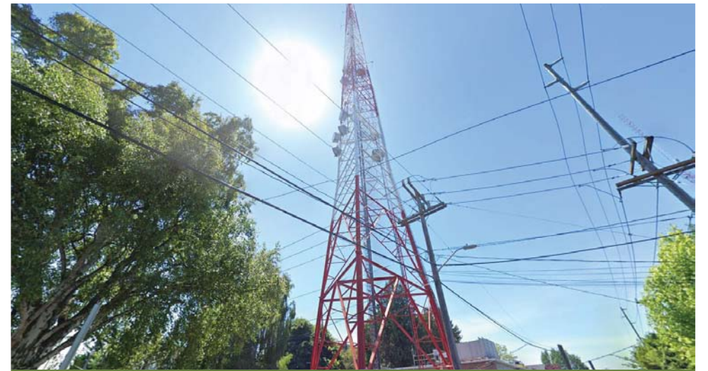
3 KOMO TV TRANSMITTERS
