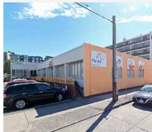
⑩ 233 6th Ave N - The Arc of King County - Office - 1 Floor
