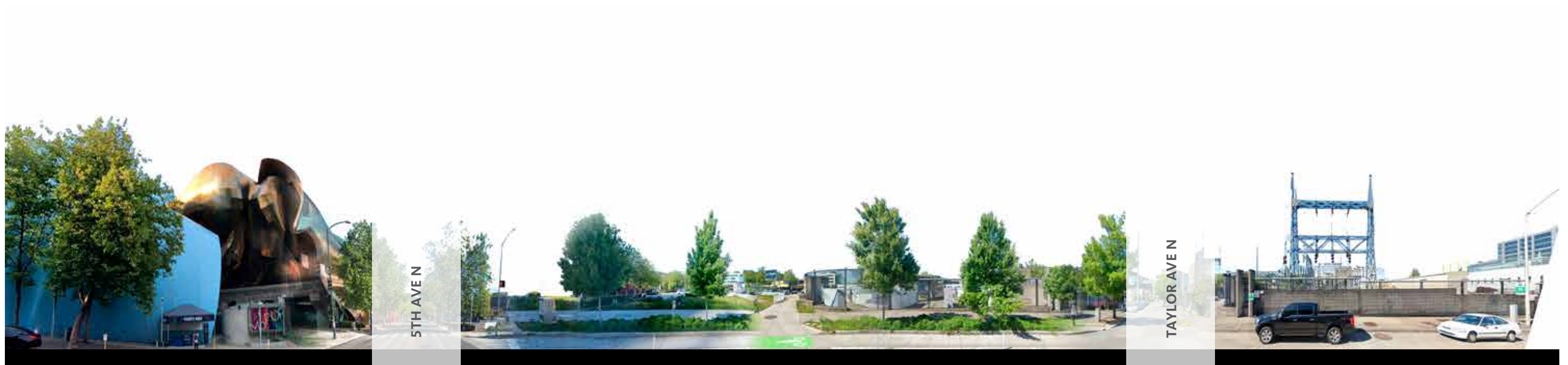
5TH AVENUE NORTH, FACING WEST
