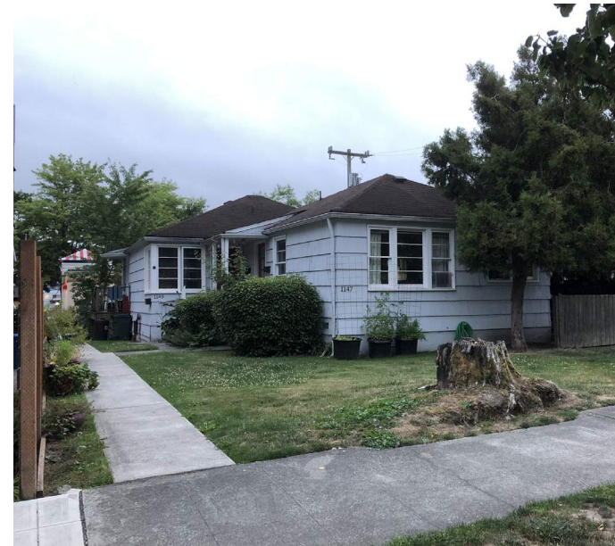
2 NORTH-EAST CORNER OF SITE
