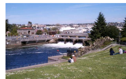
8 BALLARD LOCKS 0.8 MILES FROM SITE
