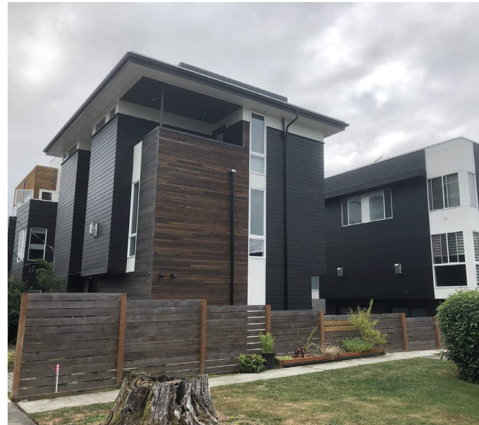
1 NEIGHBORING BUILDING EAST OF SITE FROM NW 56TH STREET
