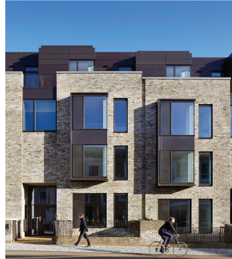
PL1.B.1 pedestrian entries through the lot are clearly marked but inconspicuous, focusing on the facade as a whole.
