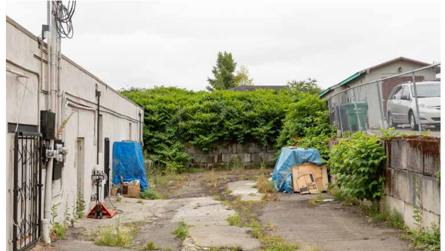
B - BLOCK RETAINING WALL ON NORTH PROPERTY LINE
