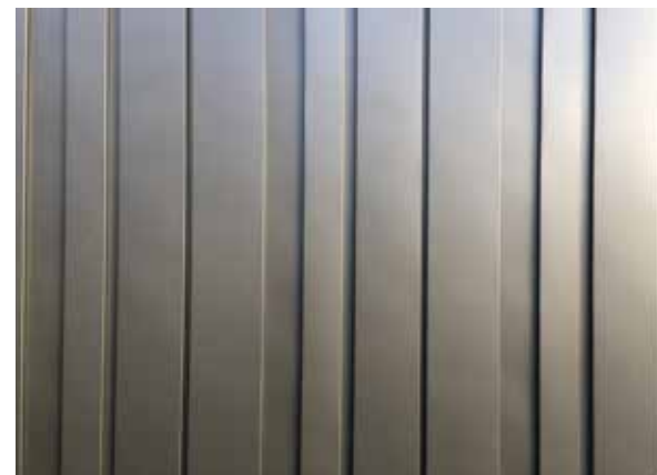
DARK GROUND LEVEL MATERIAL
