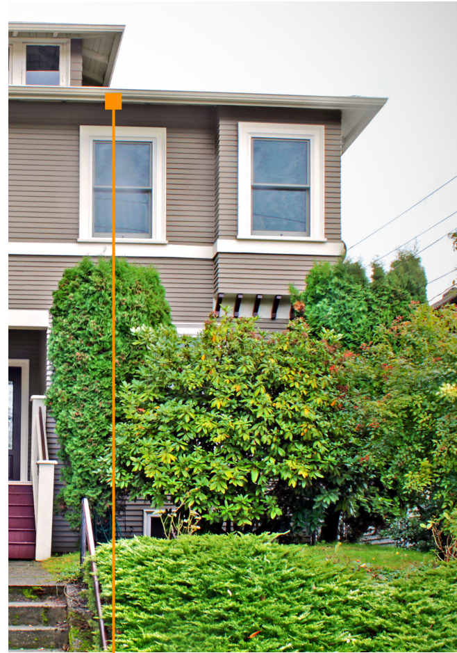
Deep eaves and low roof pitch provide a strong horizontal terminus at top of building
