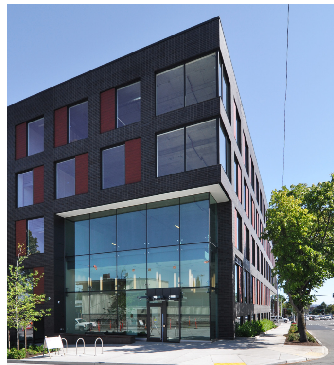
3 Office building at 15th Avenue NW and NW Market Street
