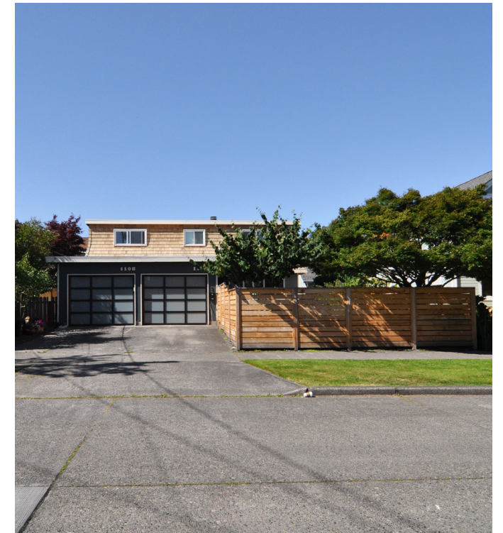
12 Single Family House on NW 57th Street between 14th Avenue NW and 11th Avenue NW
