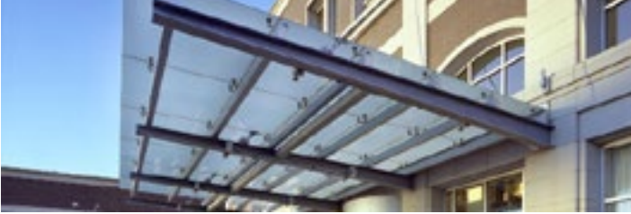
VISION GLASS WITH TUBE STEEL
