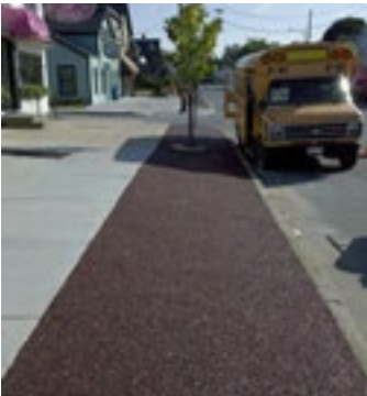
FLEXIBLE PAVING AT TREES
