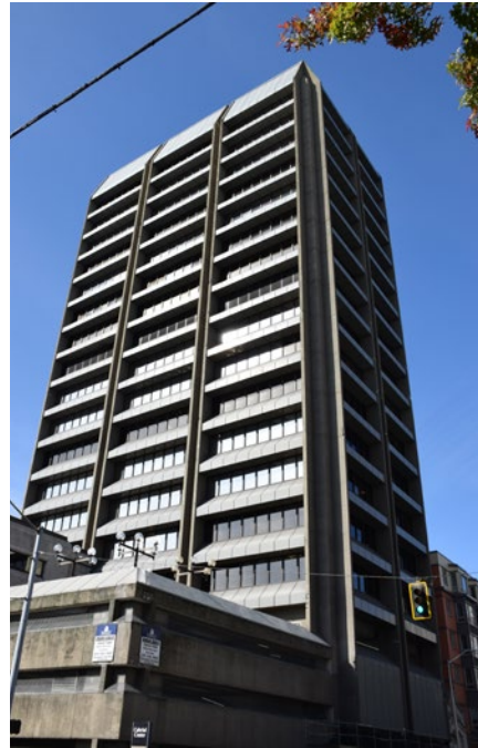
1973 / 19 Stories Medical Office Building
