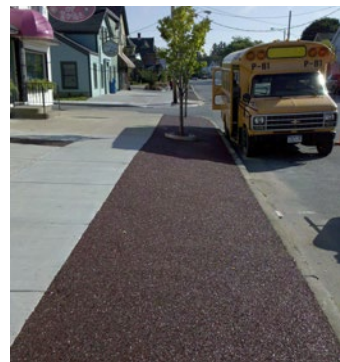
FLEXIBLE PAVING AT TREES
