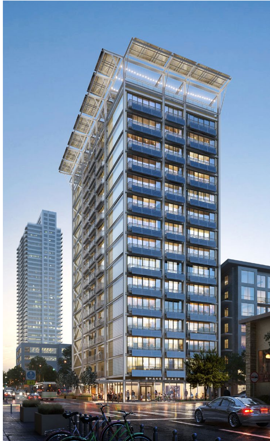
303 Battery - Seattle, WA
