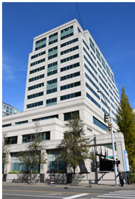
1994 / 14 Stories Medical Office Building
