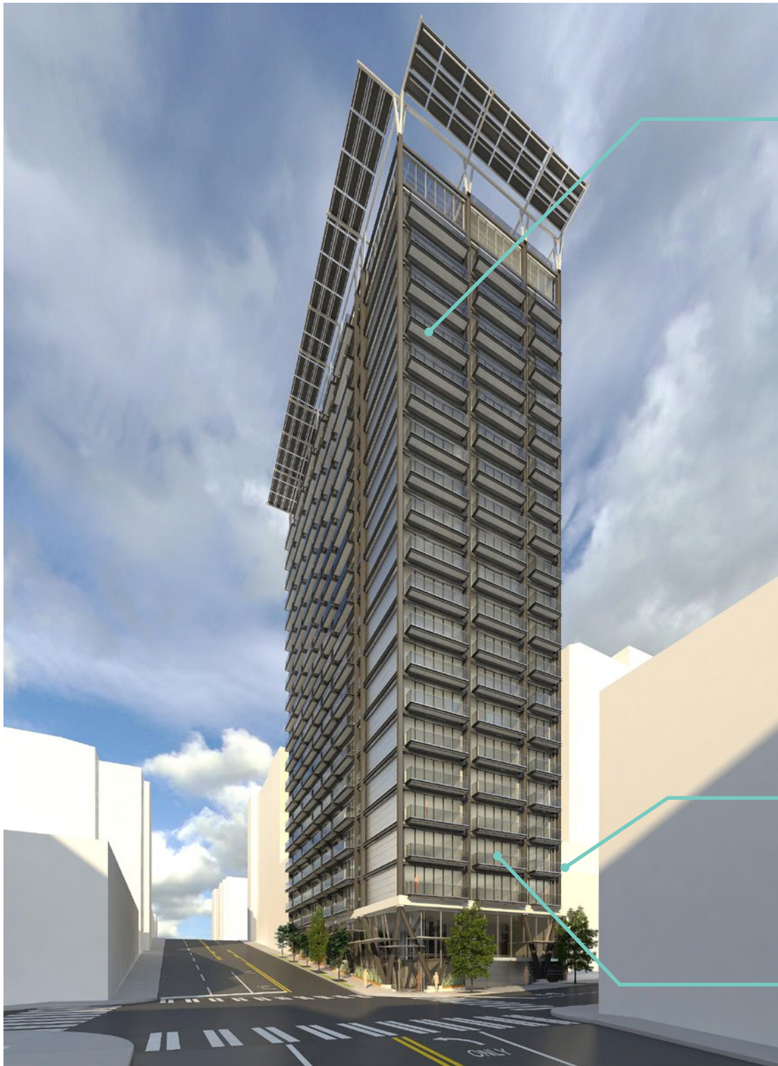
View from Madison Street and 9th Avenue
