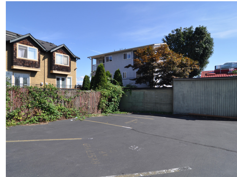
⑦ View looking Southeast at adjacent structures from site
