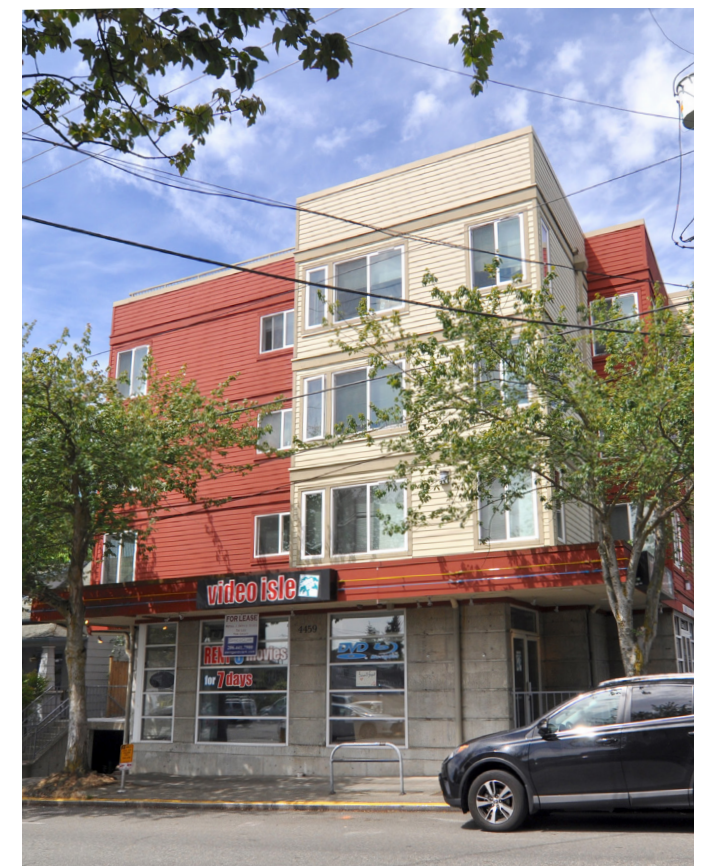
2 Mixed Use apartment along Fremont Ave N
