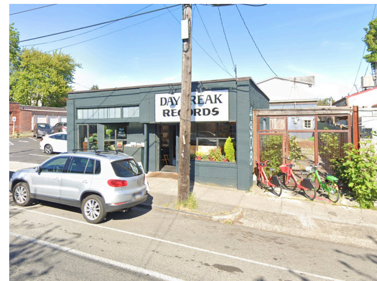
8 Commercial Store along Fremont Ave N
