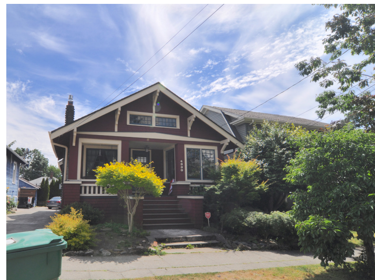
7 Single Family House on Evanston Ave N
