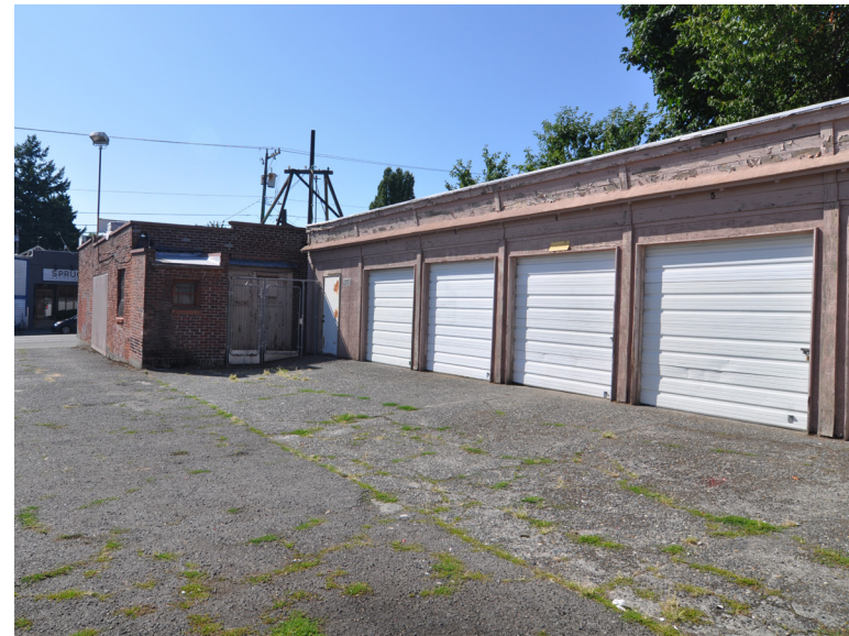
⑥ View looking West at existing structure from site
