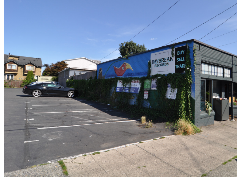
③ View looking east at adjacent structure from Fremont Avenue North
