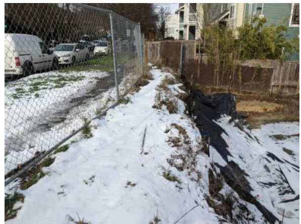
PHOTOS OF EXISTING CONDITIONS
