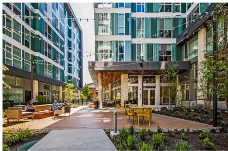
Mix of on Grade Materials
