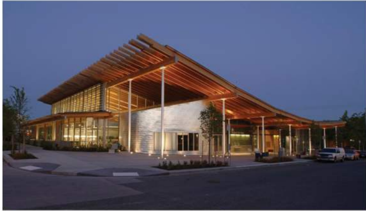
5 Ballard Branch- Seattle Public Library
