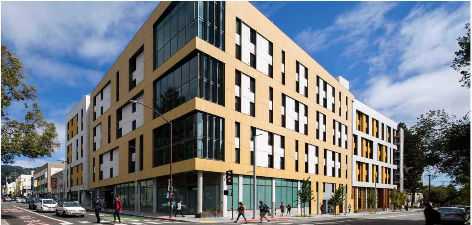
Stacked Floor Grouping of Window Patterns at Corner
