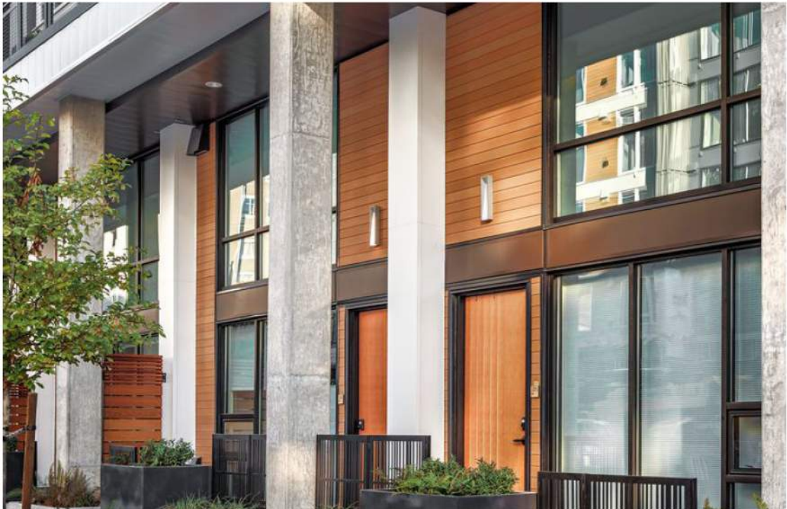
Wood Panels and Concrete
