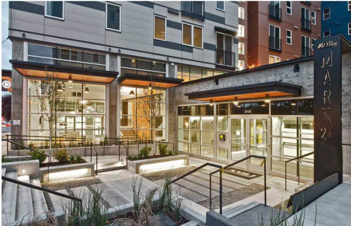
Concrete and Steel Corten
