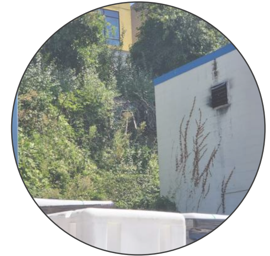
1 - RETAINING WALL AT STEEP SLOPE
