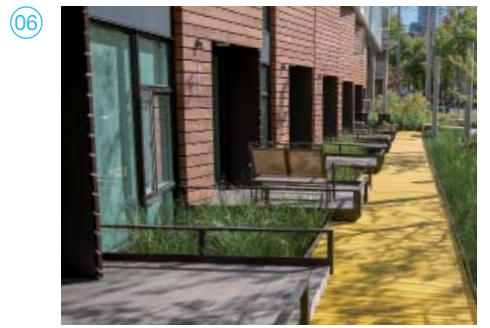
Stoops Above Bioretention Planters
