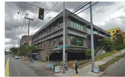
1 RETAIL | PARKING | ACCESS
