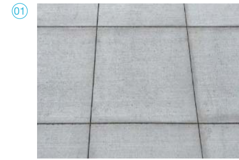
Standard 2'x2' Concrete Sidewalk
