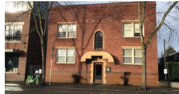
1 MASONRY - APARTMENT BUILDING
