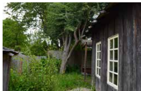
6. BACKYARD LOOKING NORTH
