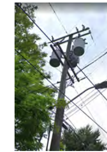
SL-1 Existing Pole mounted "Cobra head" Street Light
