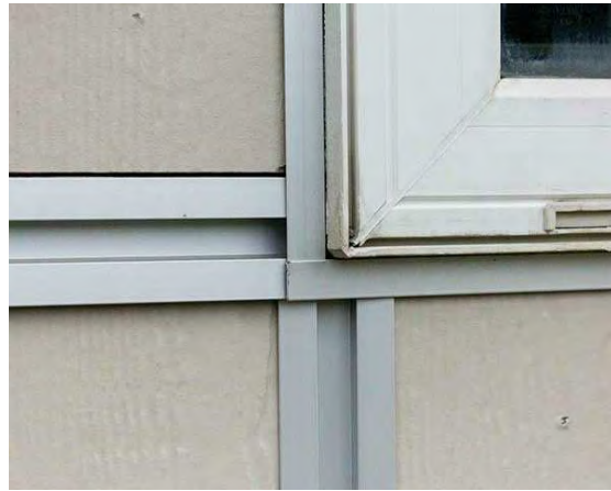
A Example of Cement Panel Window Detailing
