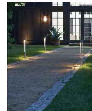
LG-1 Low Voltage Landscape Lighting at Entry Pathway
