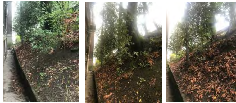
EXISTING RETAINING WALL SHOWN BOWING ON SOUTH OF SITE AND TREES OF AN INVASIVE SPECIES GROWING FROM A STEEP SLOPE.
