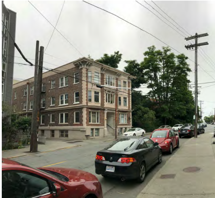
South Adjacent Structure
