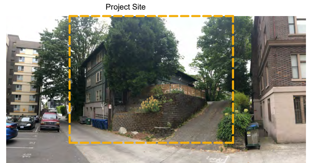
West Side of Site in Alley Looking North
