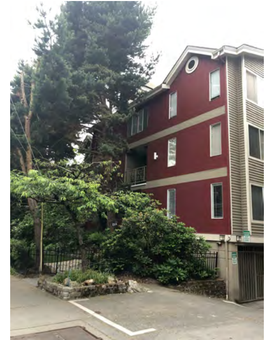
North Adjacent Structure
