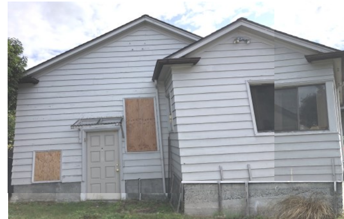
Existing House- West View
