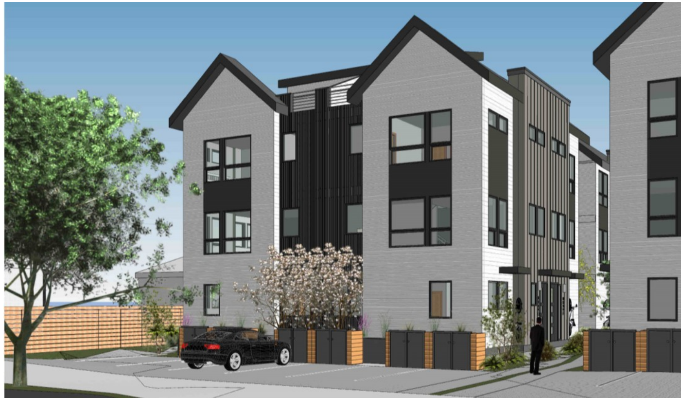
VIEW FROM SOUTHWEST
