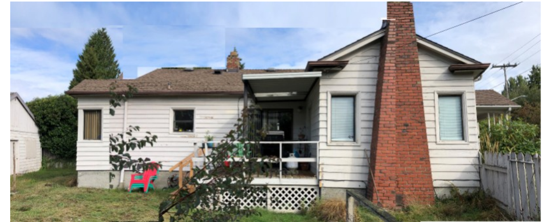
Existing House- South View
