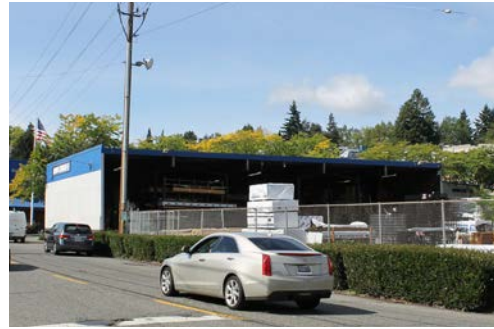
3 DUNN LUMBER YARD SHELTER
