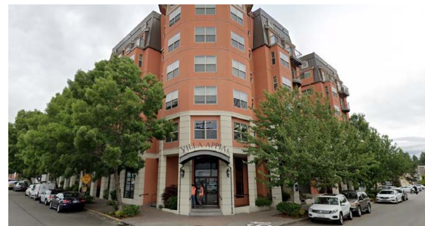
F—12300 31ST AVE NE
