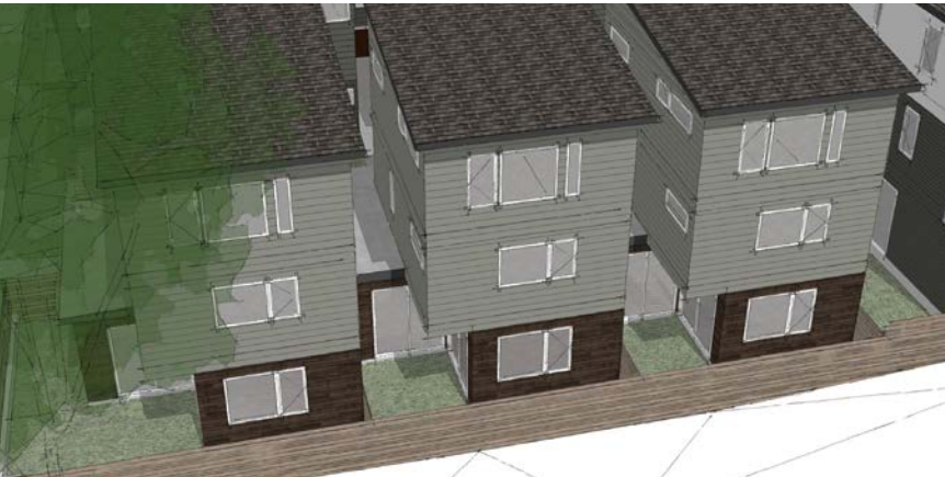
Units 6-8 have south facing yards carved out of the first floor with a deep overhang above part of the yard to provide weather protection and shading at different times of year. The living space is designed with large patio doors to provide a strong visual connection between indoor and outdoor spaces.
