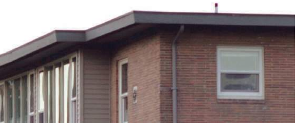
In a typical project, stormwater is directed from roof to gutters and downspouts then to a storm drain or a combined sewer/storm drain.
