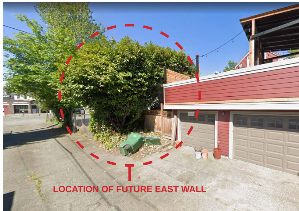
Existing Neighboring Condition @ East Wall
