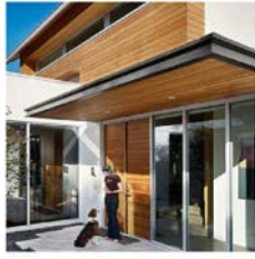
Canopy - Steel Channel/Wood Soffit
