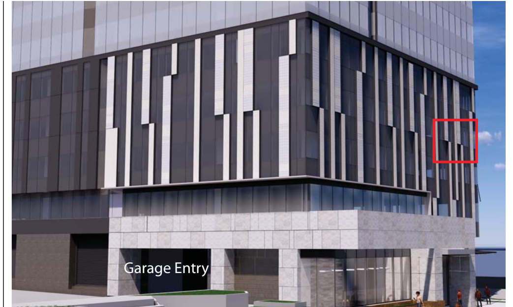
Terracotta and Stone wrap around to alley
