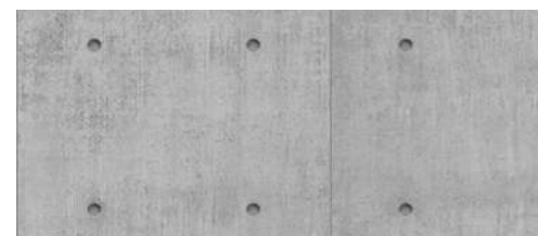
⑦ CAST-IN-PLACE CONCRETE SMOOTH FINISH
