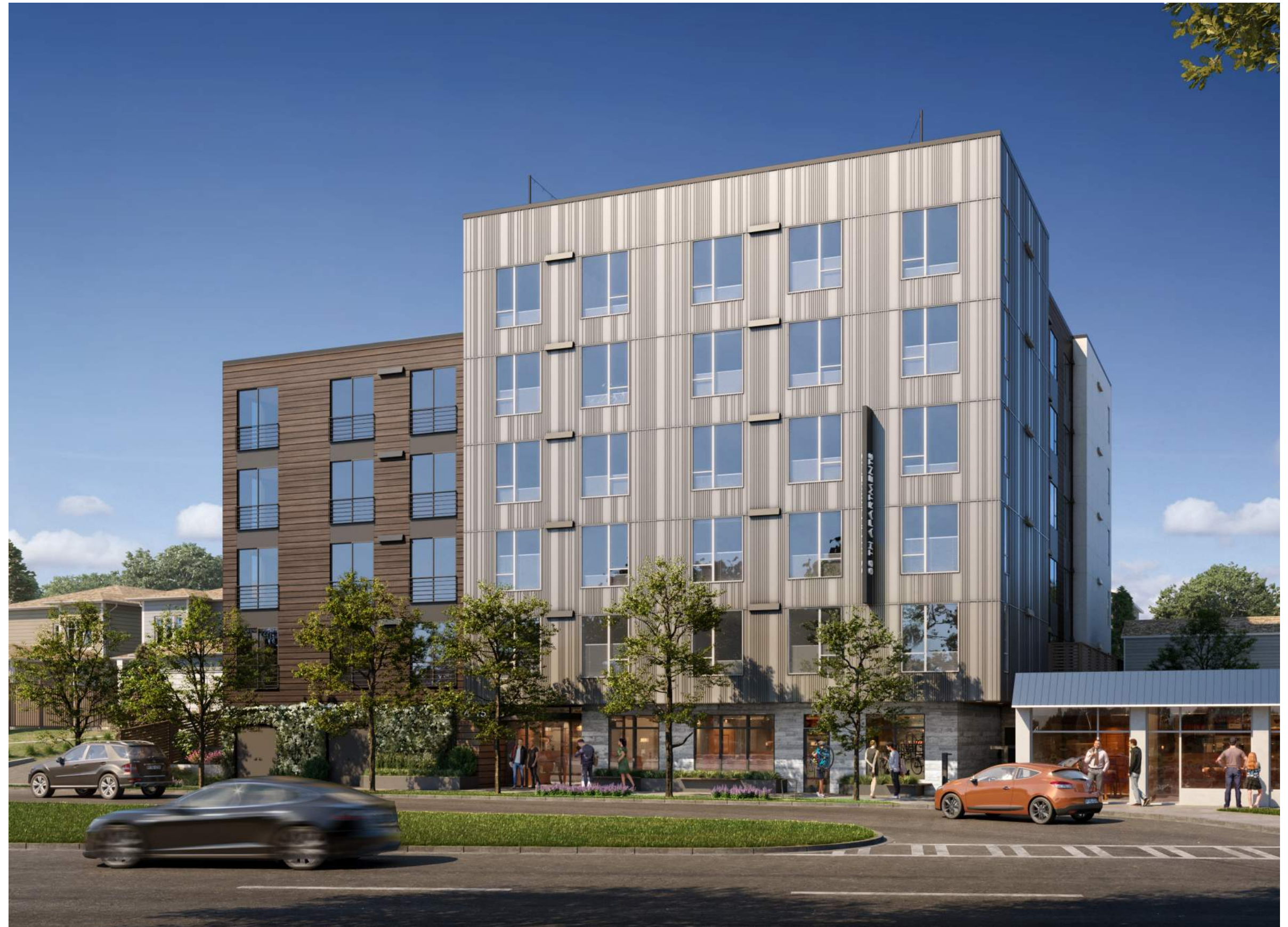
VIEW OF NORTHEAST CORNER
