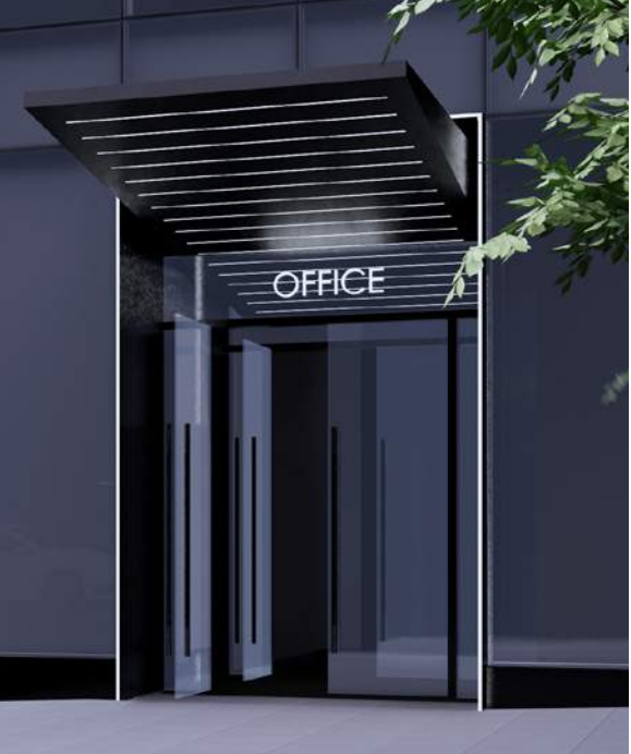
RECESSED LINEAR LENSED FIXTURE AT OFFICE CANOPY
