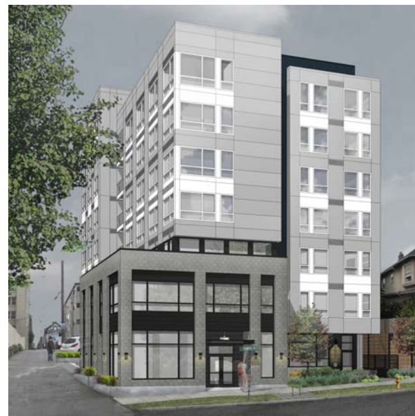
600 E Howell St (Under Construction)
