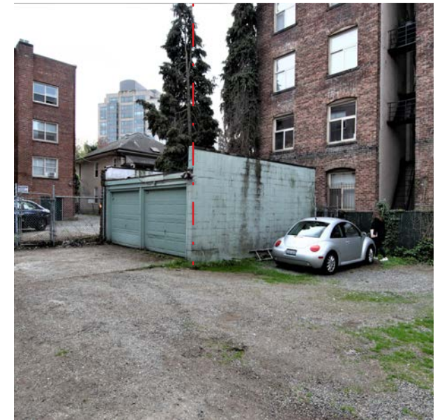
Looking at southwest property corner
