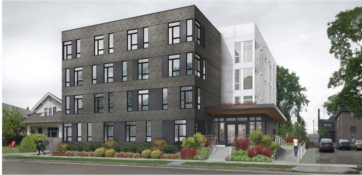
4710 20th Ave NE (Under Construction)
