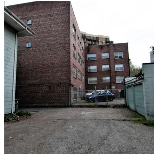
Looking at south neighbor
