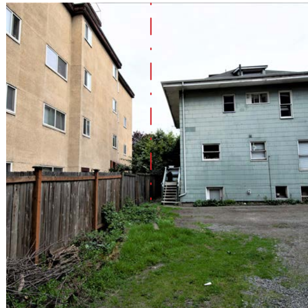
North property line looking east
