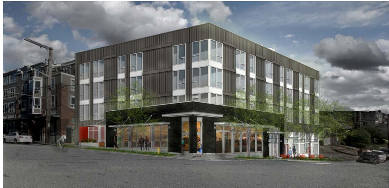
800 5th Ave N (Under Construction)
