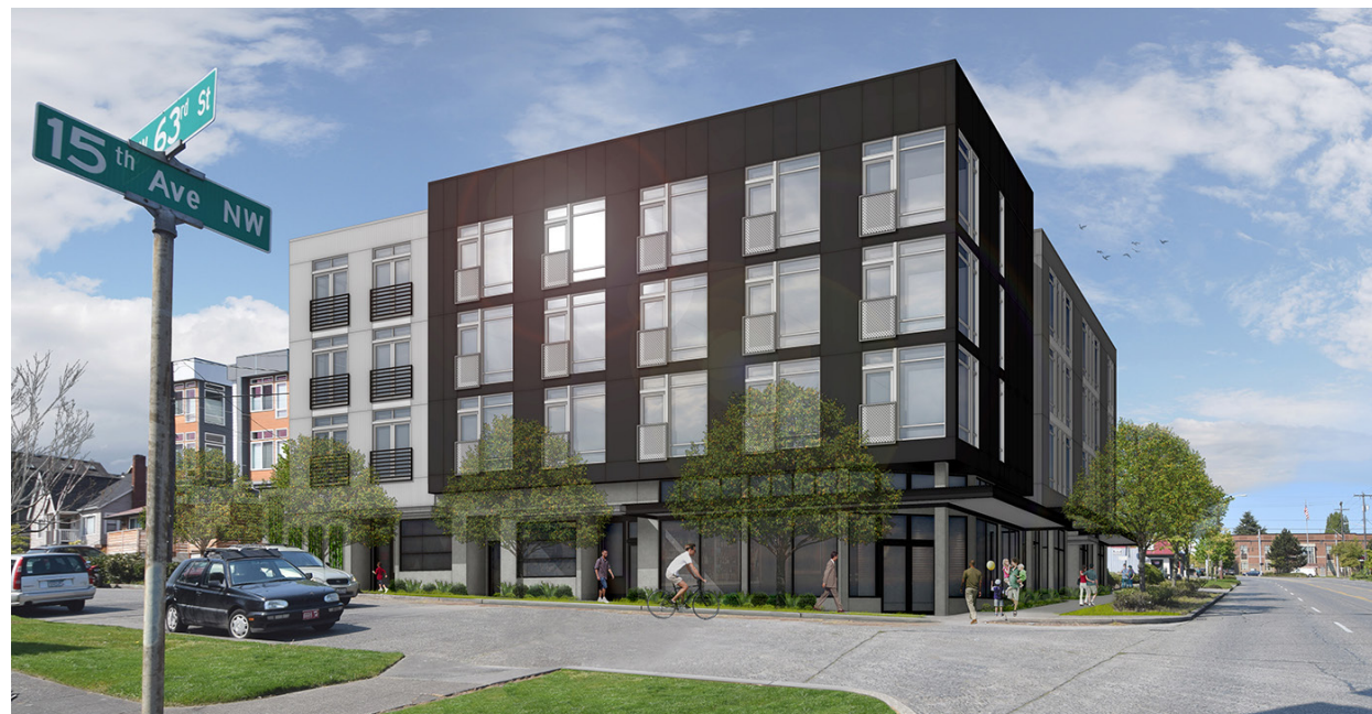
6301 15th Ave NW (Under Construction)
