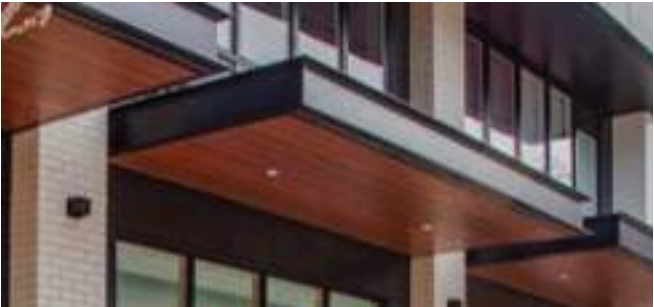
Metal frame canopy with wood soffit. Canopy raised to signify entry
