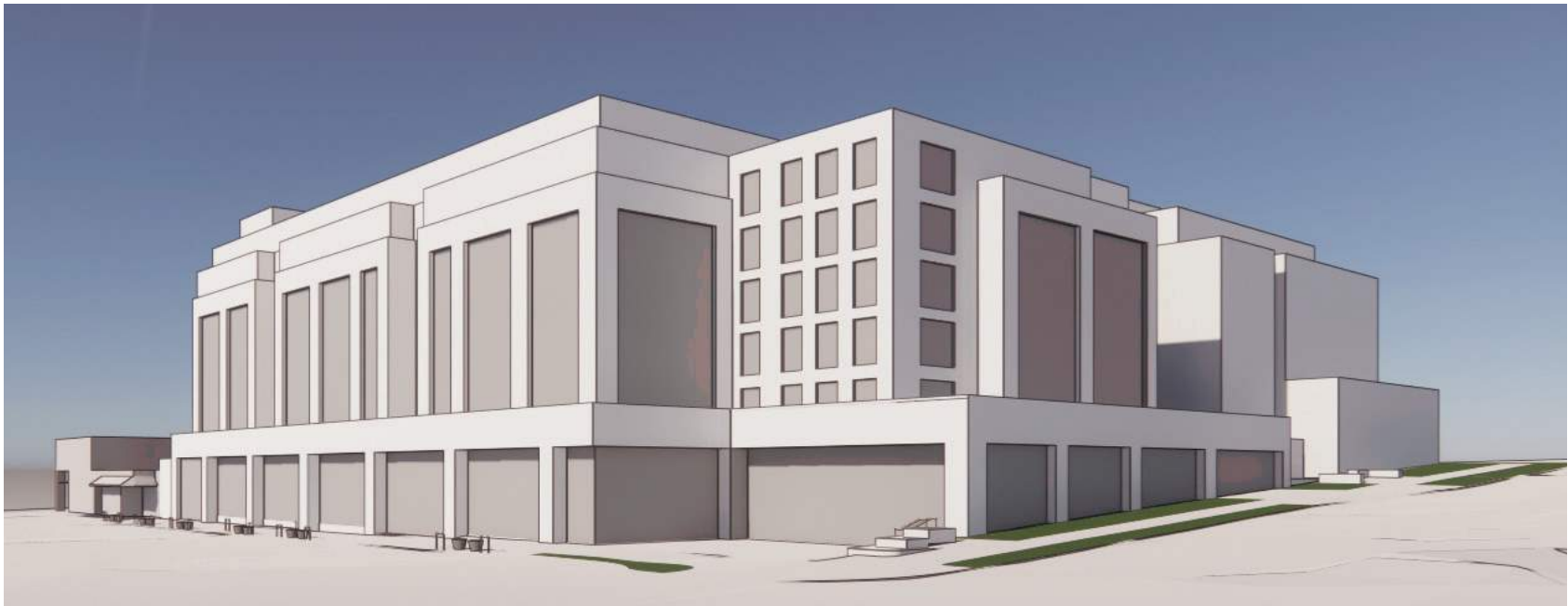
Building C massing refinement: the plinth evolves as a brick base with retail bays. On the upper floors, a corner element with punched openings contrasts with brick bays with metal infill.
