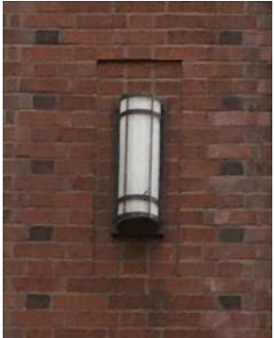
Example - Recessed soldier course at light fixture
