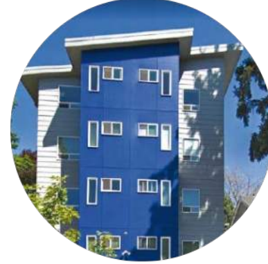
3 Shed roof at multi-family housings
