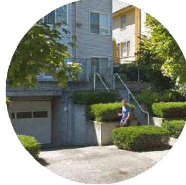
2 Stepped planters with stair to residential level at a multi-family housing
