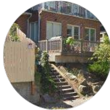
5 Elevated deck facing street
