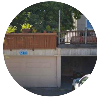
1 Garage access from street, patio on top of garage
