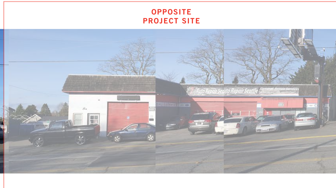
1 Story commercial building
