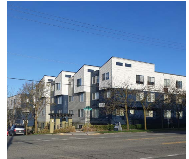
3 10301 GREENWOOD AVE - Color variation to create interest in the exterior facade.
