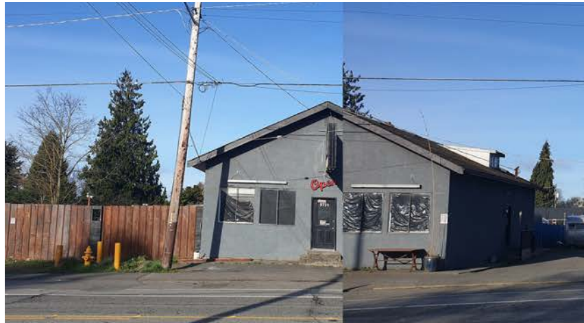
1 Story commercial building
