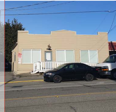
1 Story commercial building
