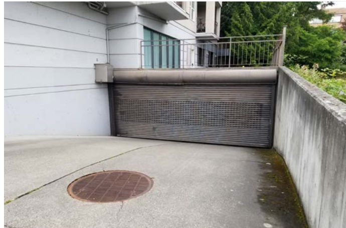
4 DRIVEWAY FOR ADJACENT PROPERTY TO THE NORTH
