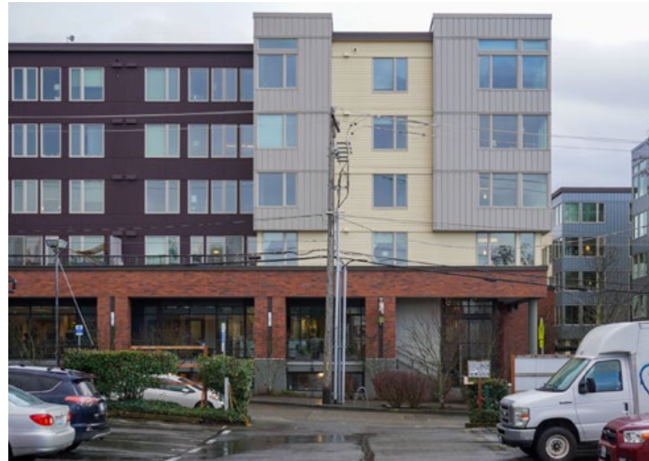
14 Looking South across NE 72nd to GreenLake Village from the existing surface parking lot on the project site.
