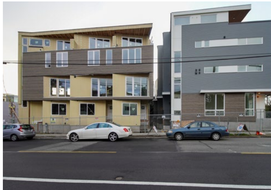
04 Looking West at newly constructed 4-story residential project at corner of NE 73rd St and 5th Avenue NE. Project site is to the left of this photo. 01.26.20.
