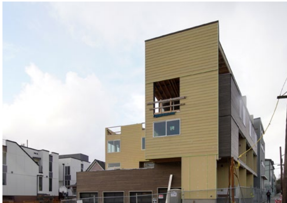
05 Looking North at newly constructed 4-story residential project at corner of NE 73rd St and 5th Avenue NE. Project site is to the left of this photo. 01.26.20.
