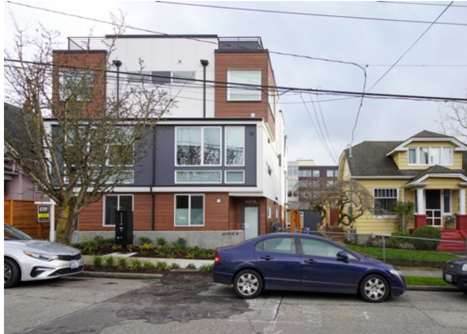
02 Looking South at newer construction of two in-line 3-story residential buildings (left) and an existing 2 level single-family detached
