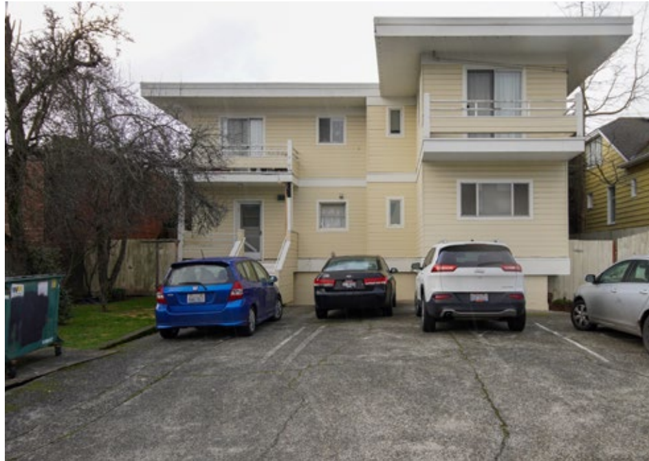
07 Looking North from mid-block alley to newer construction of a 2-story residential project with surface parking at rear (alley-side) yard. 01.26.20.
