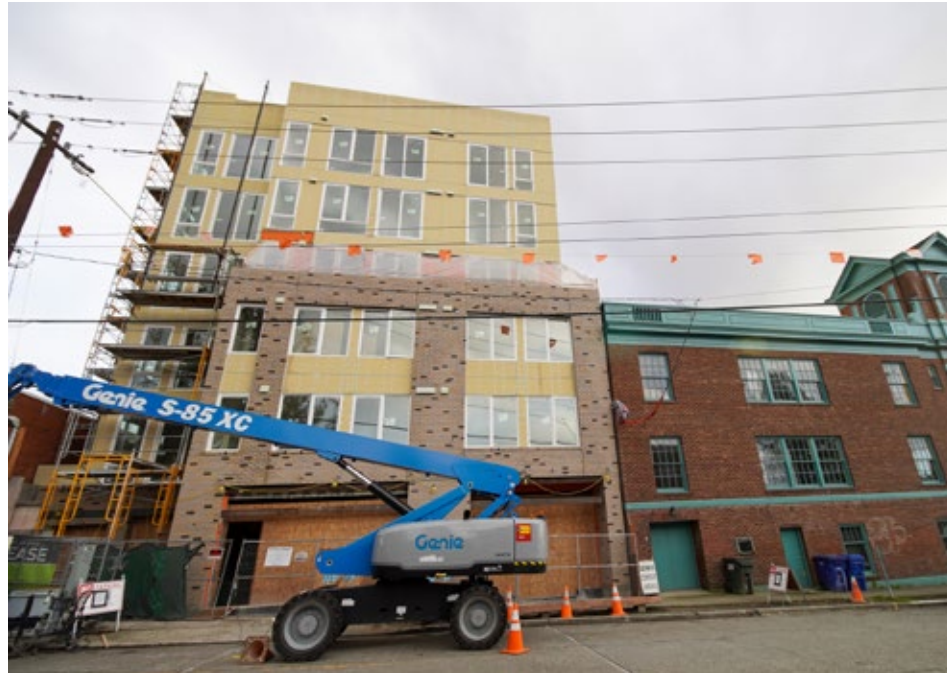
01 New 6-story residential project along west end of NE 73rd Street adjacent to Great Hall at Greenlake. 01.26.20.
