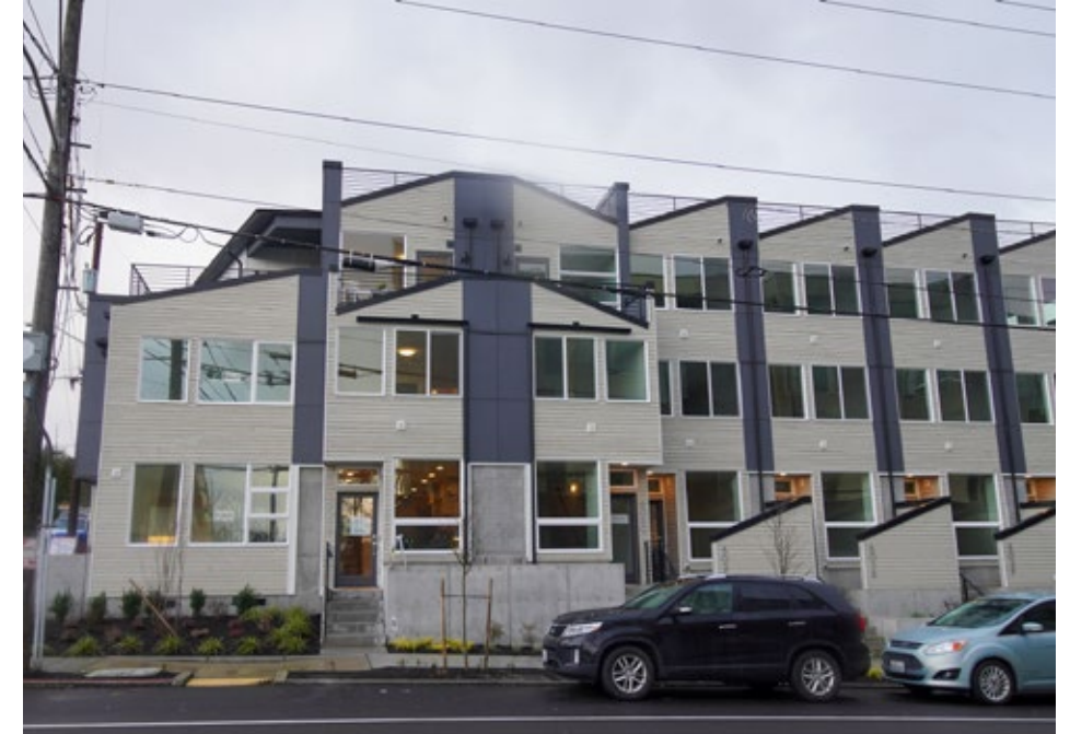
15 Looking South across NE 72nd to GreenLake Village from the existing surface parking lot on the project site.
