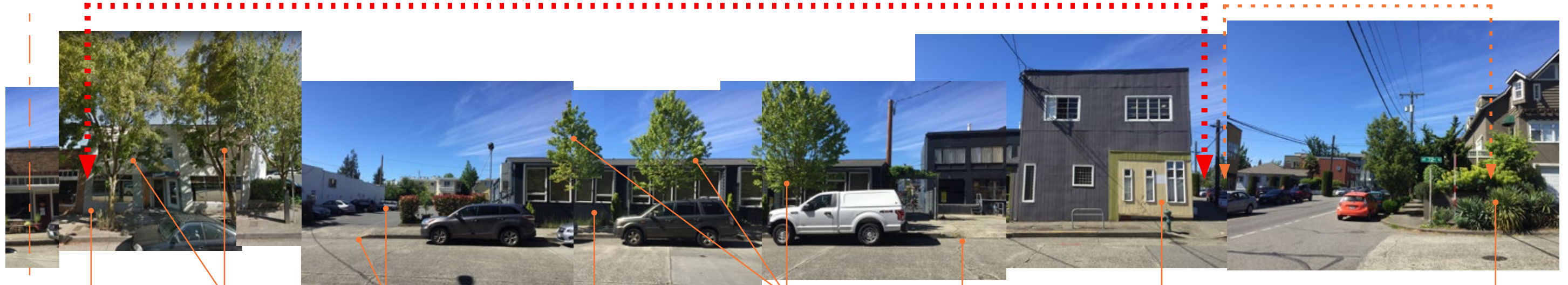
Existing office building "Vitamilk" (to be removed)
