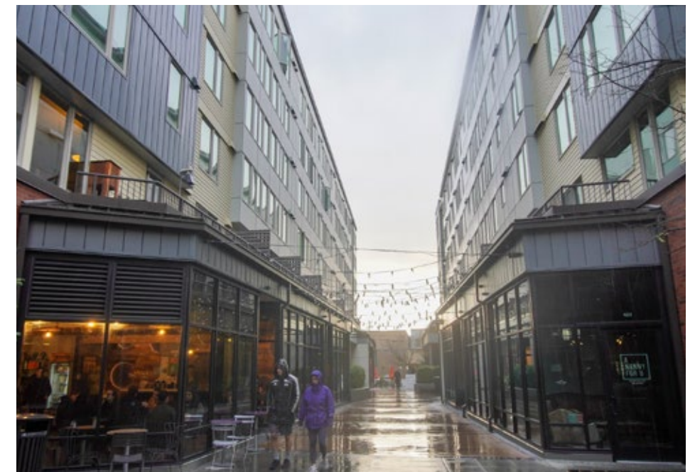
12 Looking West between 2 of the buildings at GreenLake Village along the internal pedestrian street.
