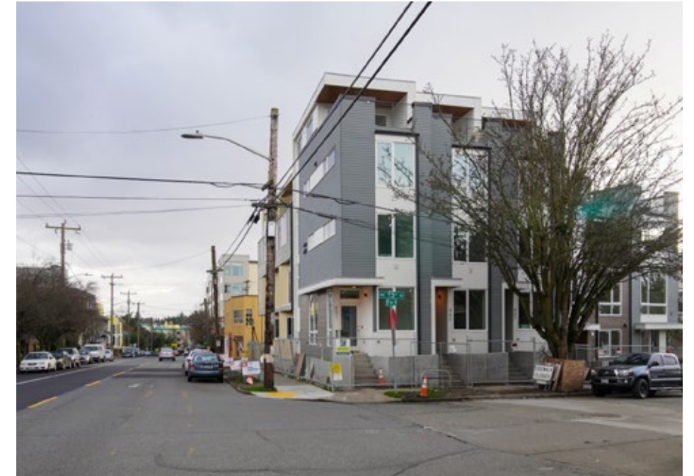
03 Looking South at newly constructed 4-story residential project at corner of NE 73rd St and 5th Avenue NE. 01.26.20.
