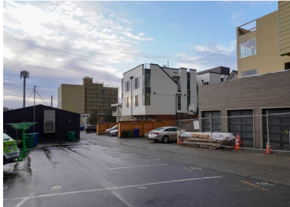
08 Looking northwest along alley from the existing surface parking lot on the project site. of a 2-story residential project with surface parking at rear (alley-side) yard. 01.26.20.
