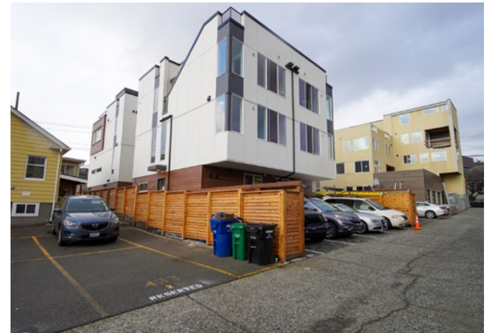
06 Looking NorthEast from midblock alley at newer construction of two in-line 3-story residential buildings. 01.26.20.
