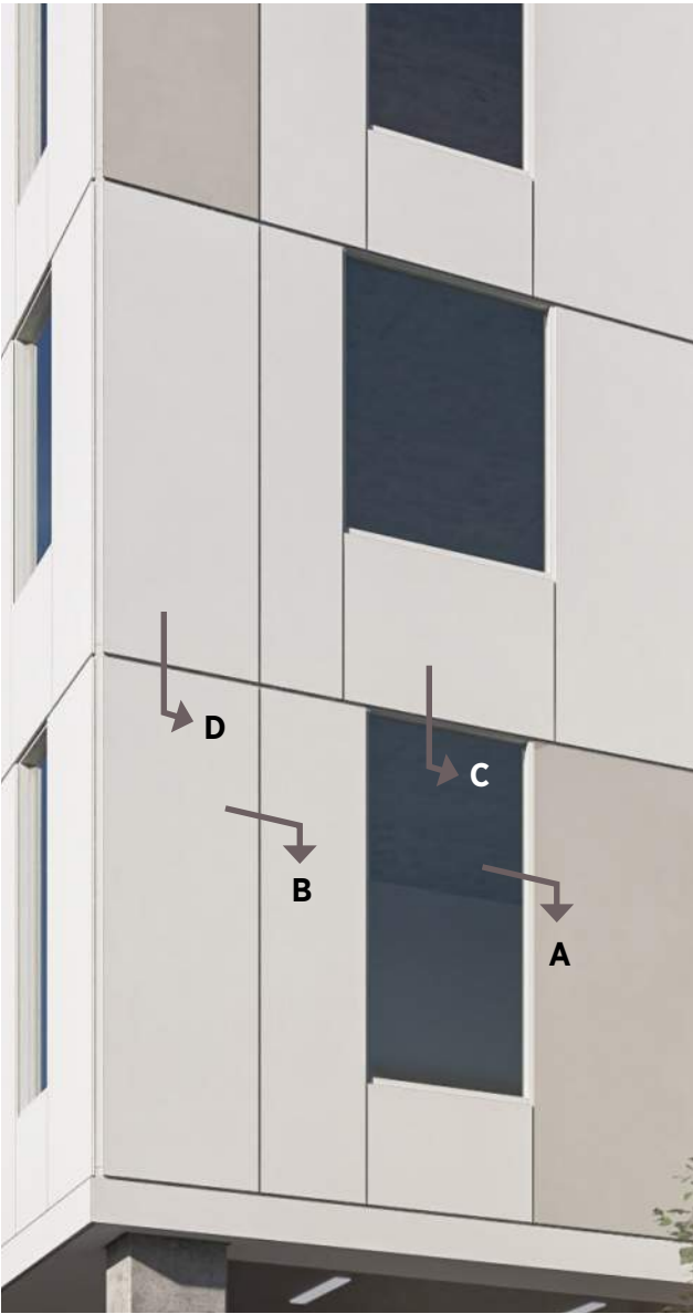
Projected metal panels cover mullions and floor slabs for refined appearance. This flush appearance will be in contrast with the depth of the Connector. Depth and interest is in the form of color and shape variation and in the contrast between opaque and clear wall.
