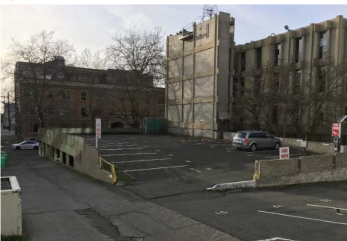
G ALLEY LOOKING SOUTH
