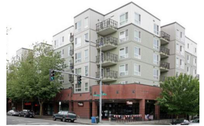
3 Towers on Greenwood - 8551 Greenwood Ave N - 70 units
