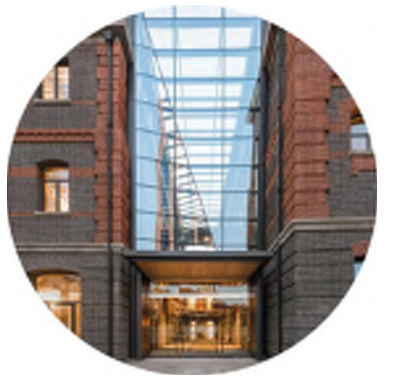
6 Transparent gasket and residential entrance between brick facades
