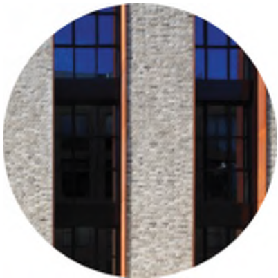
1 Brick to infill transition detail
