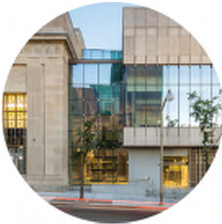
3 Transparent gasket creates separation between the historic and new development
