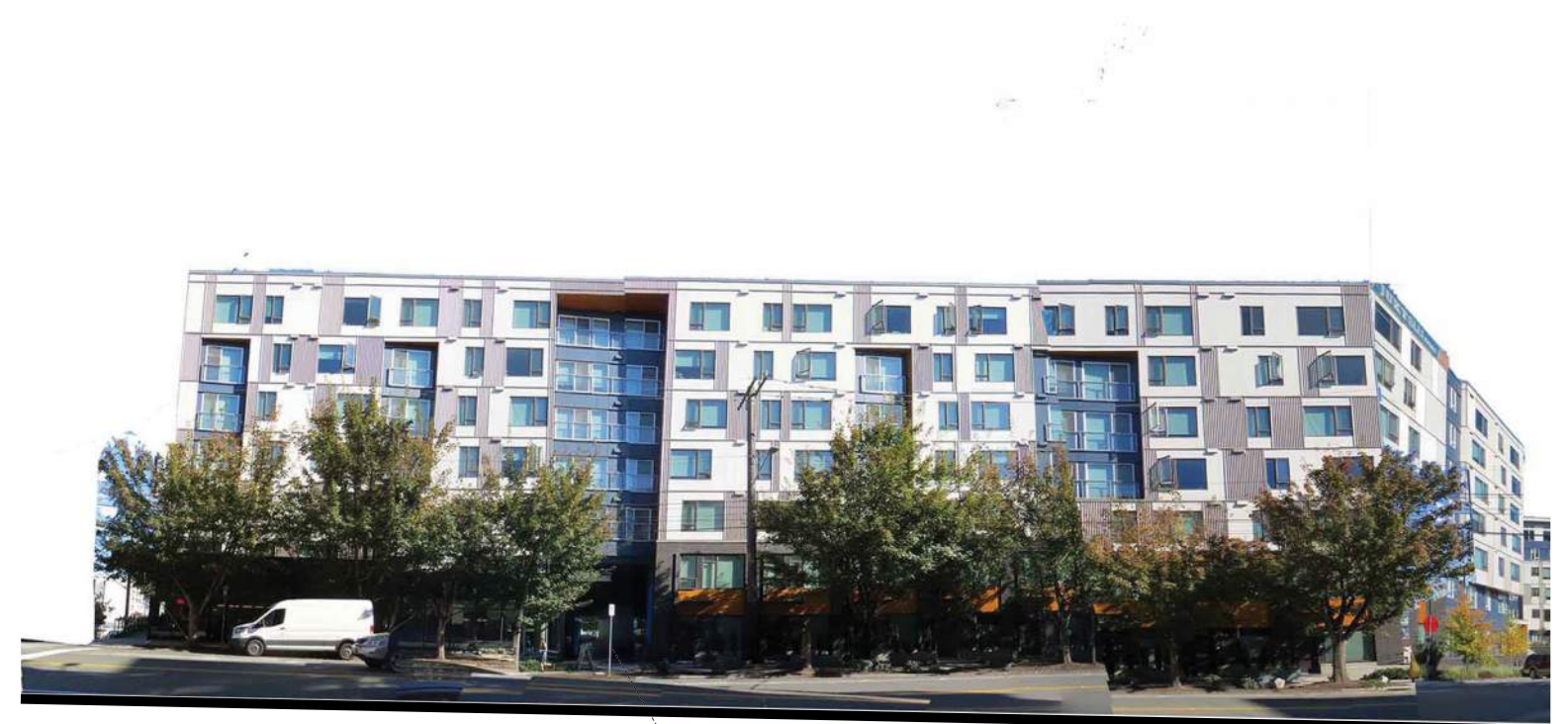
B - VIEW LOOKING EAST ON DEXTER AVE N
