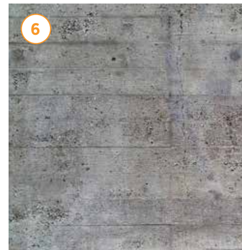
BOARD FORMED CONCRETE
