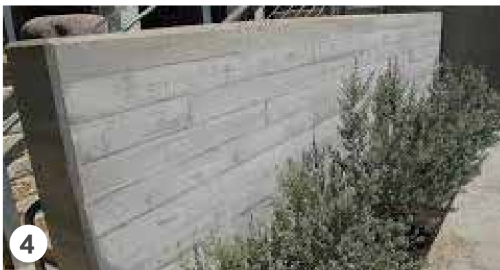
BOARDFORM CONCRETE WALL
