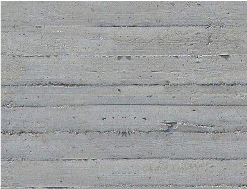
BOARD FORMED CONCRETE (AT SIDEWALK RETAIL BASE)
