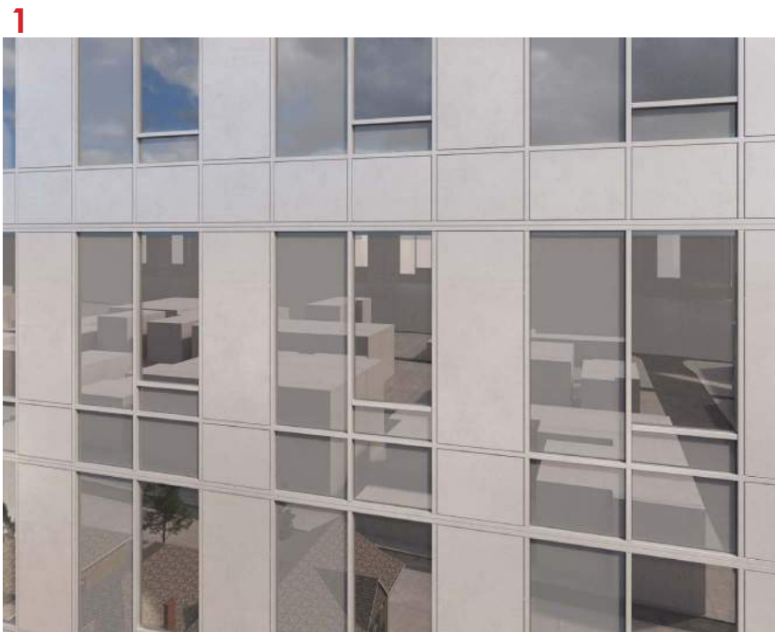
WINDOW WALL - METAL PANEL, SPANDREL, GLASS
