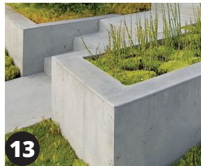
13 CAST IN PLACE CONCRETE PLANTERS
