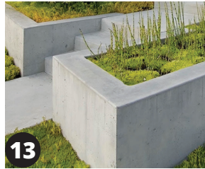
13 CAST IN PLACE CONCRETE PLANTERS
