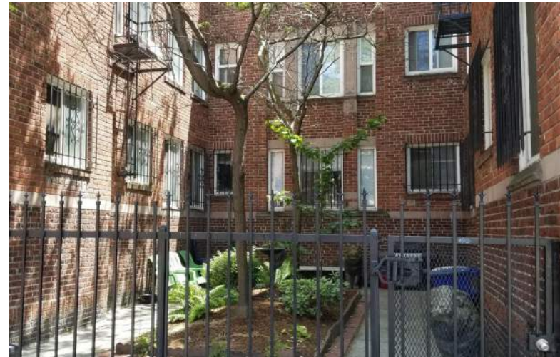
Charlesgate Apartment. : Gated courtyard is not contributing to public
