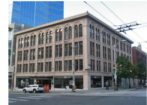
5. Doyle Building, 119 East Pine St. - Designated Landmark
