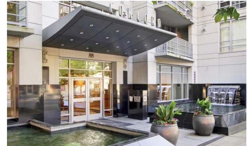
CONCORD CONDOS: Blocked off by oversized water features
