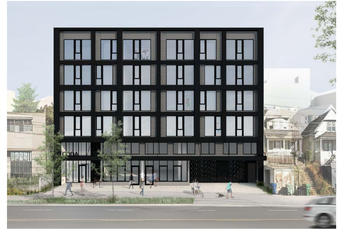
Workshop AD, KKLA, & Umtanum Build | CODA mixed-use | Seattle WA
