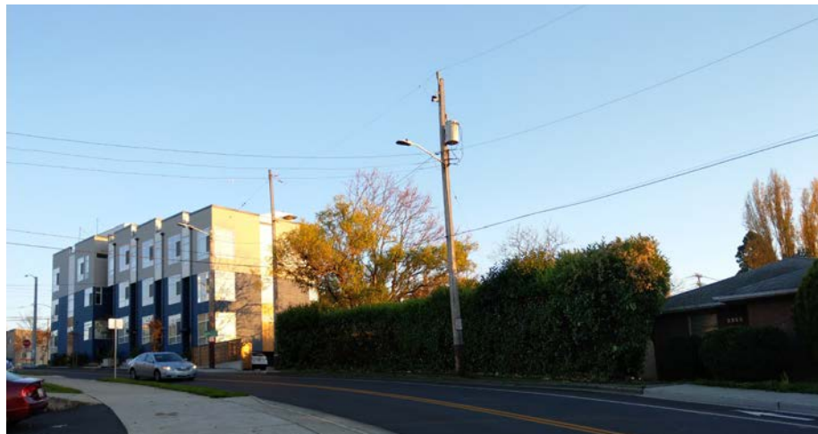
D VIEW FROM BEACON AVE S TO NORTH
