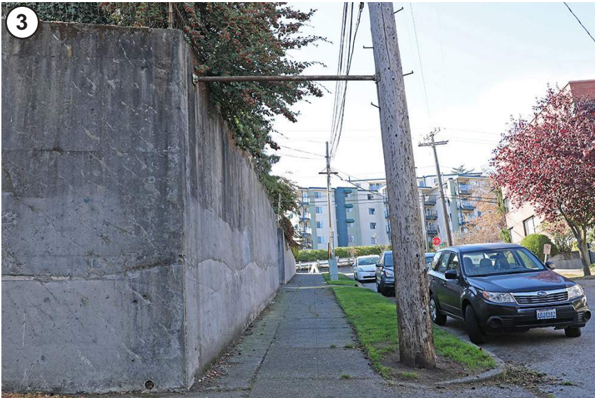
VIEW OF WHEELER POLE SUPPORT TO RETAINING WALL
