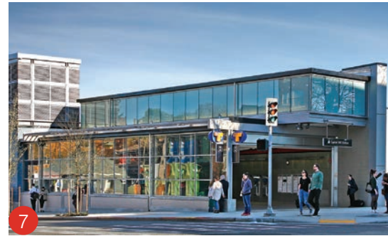
7 Capitol Hill Station
