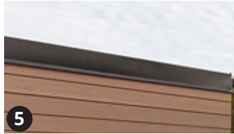
METAL CAP FLASHING, BLACK
