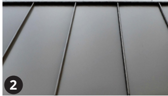
STANDING SEAM METAL SIDING
