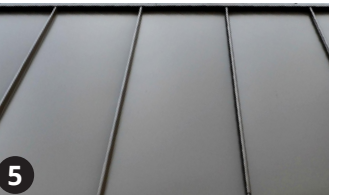
STANDING SEAM METAL SIDING
