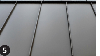
STANDING SEAM METAL SIDING
