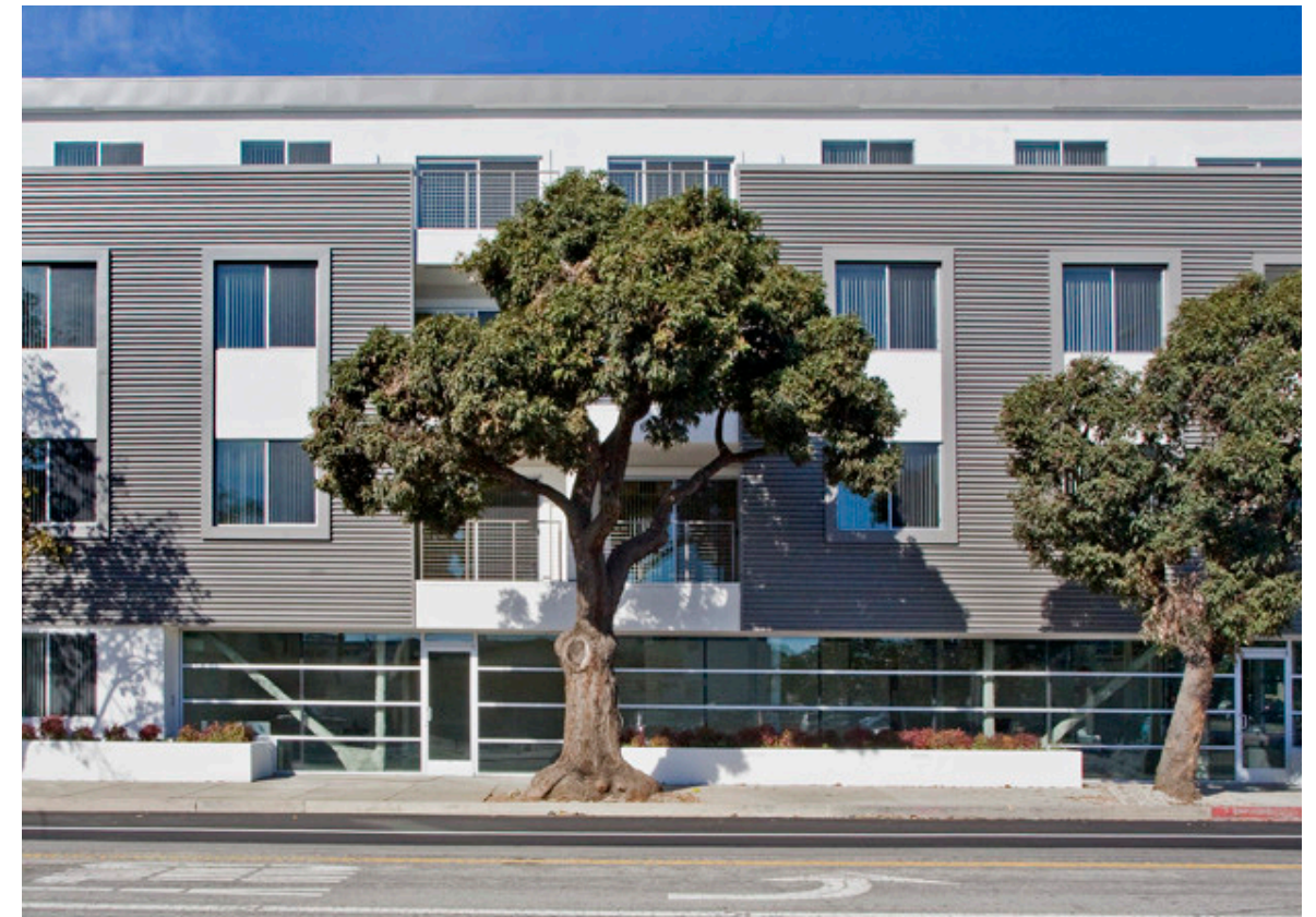
CANTILEVERED CORRUGATED METAL SURFACE
