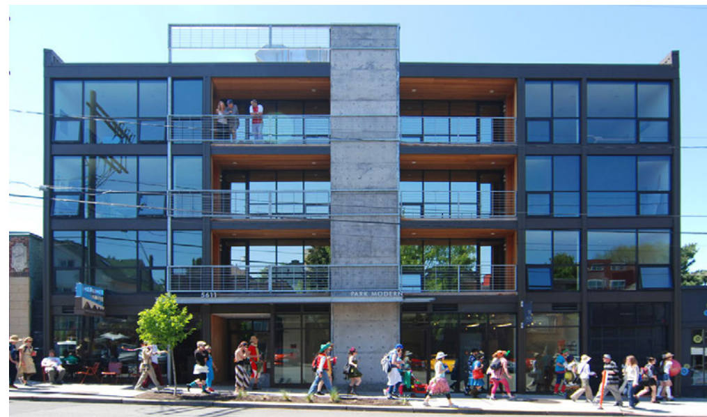
PARK MODERN - DIFFERENTIATING THE FACADE WITH MATERIAL, COLOR AND VOLUME
