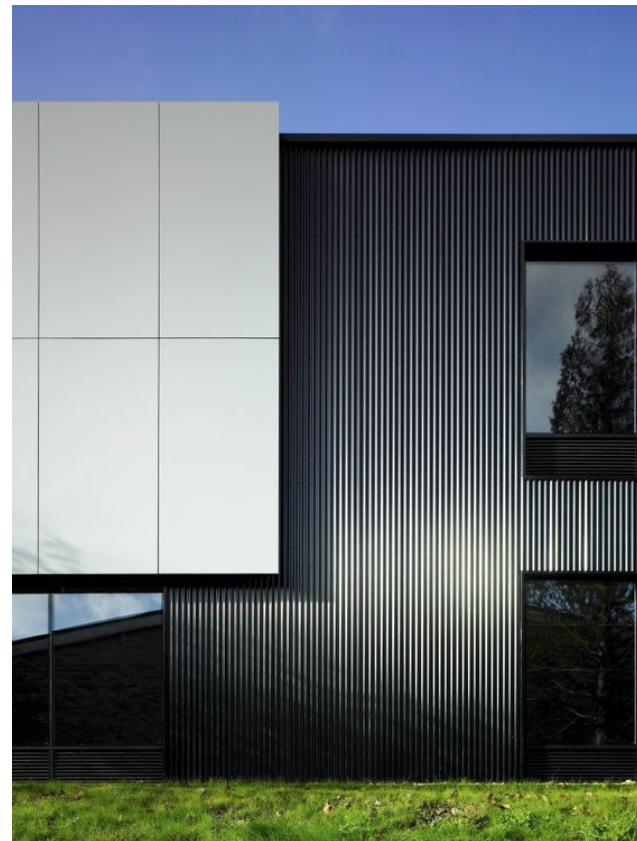
FIBER CEMENT PANEL AND CORRUGATED METAL
